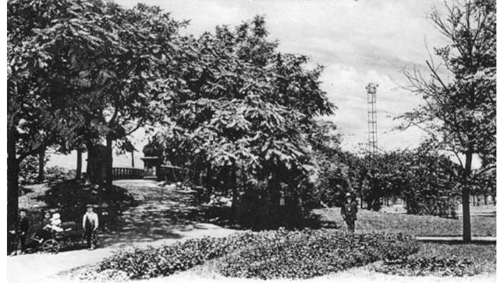
ORIGINAL WESTERN APPROACH to the pedestrian bridge over the railroad in the West Commons
