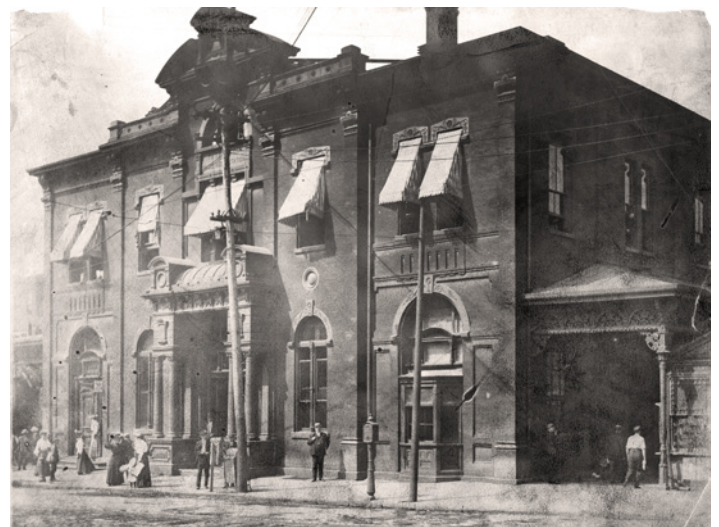
The old Fort Wayne Railroad station on Federal Street where Lincoln arrived on 14 February 1861
